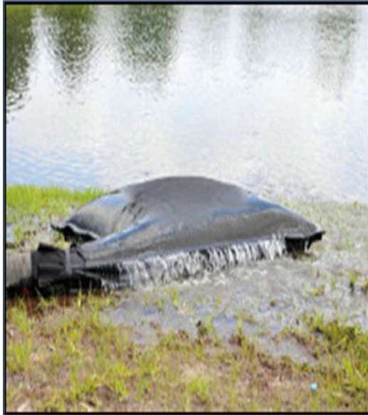
Plate 3-1. Silt Bag with water being pumped through.
