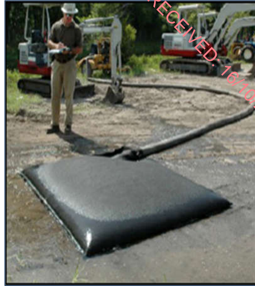
Plate 3-2. Silt Bag under inspection.
